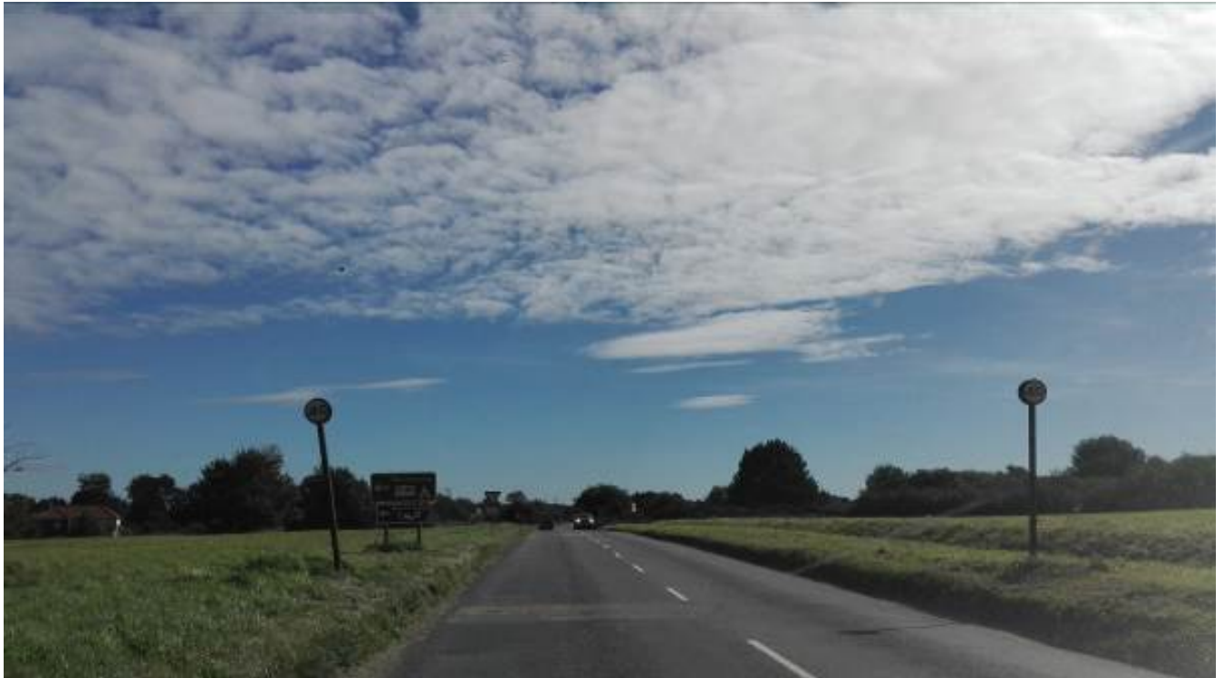
Junction approach, C550 Hempton Green Road
