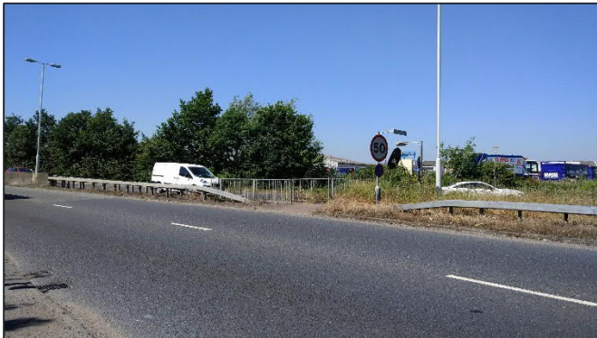
Informal pedestrian crossing facilities across the A47
