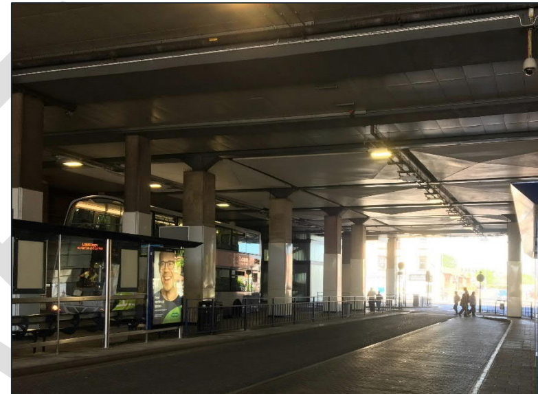
Market Gates Bus Station
