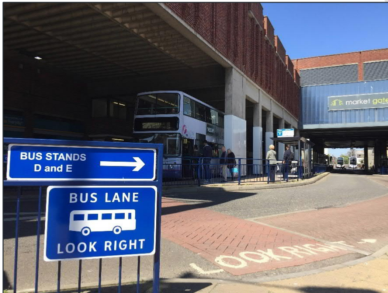
Market Gates Bus Station
